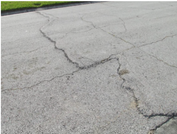
Asphalt pavement with severe transverse cracks and upheaval
