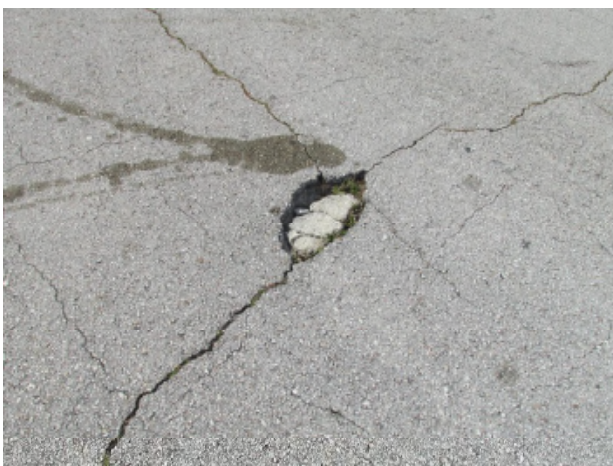
Asphalt pavement with pot hole
