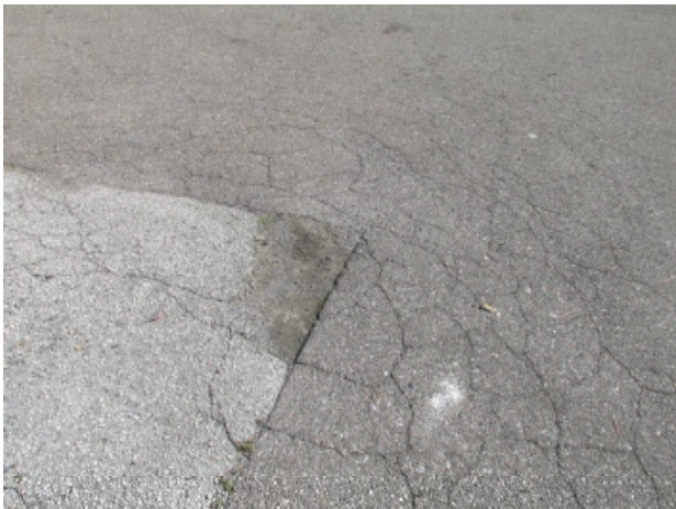
Asphalt pavement with alligator cracks
