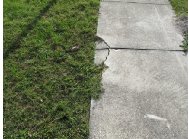
Concrete sidewalk with cracks
