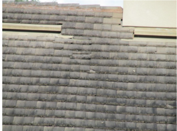
Concrete tile roof with broken tiles
