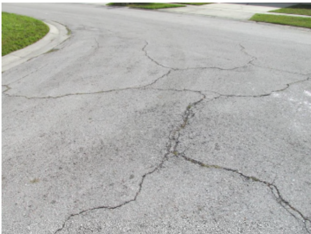
Asphalt pavement with block cracks
