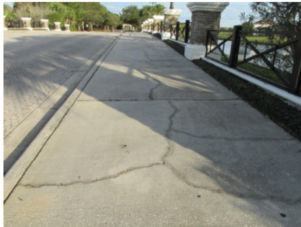
Concrete sidewalk with cracks
