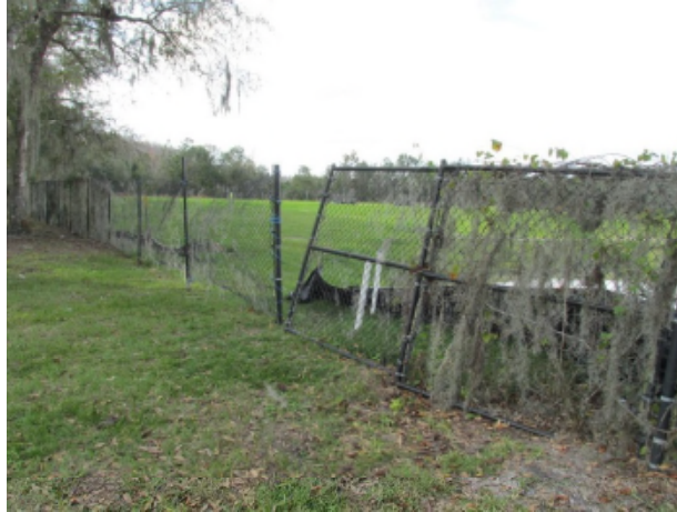
Chain link fence with lean evident
