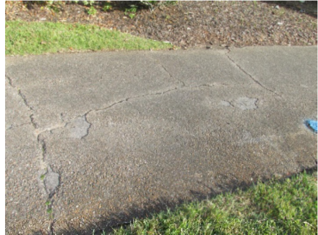
Asphalt pavement walkway with block cracks
