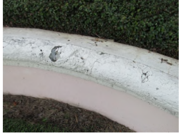
Coping damage at entrance signage
