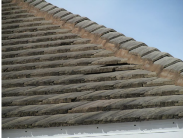
Concrete tile roof with loose tiles
