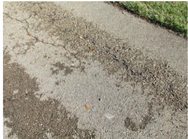
Asphalt walking path with surface deterioration
