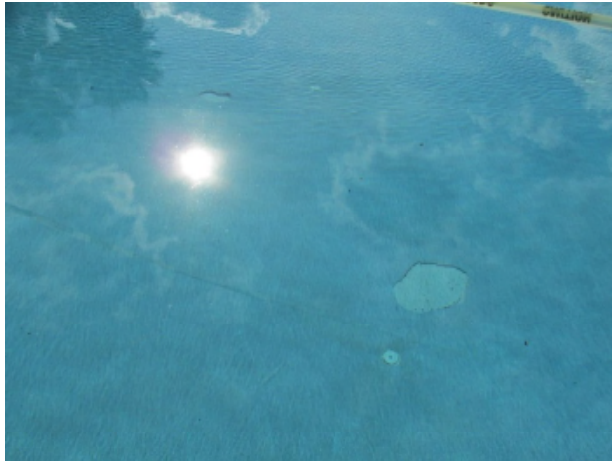
Missing plaster evident
