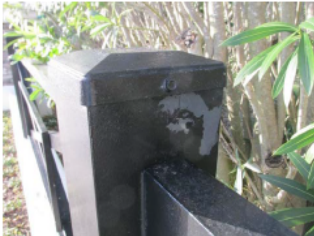
Finish deterioration at bridge railing
