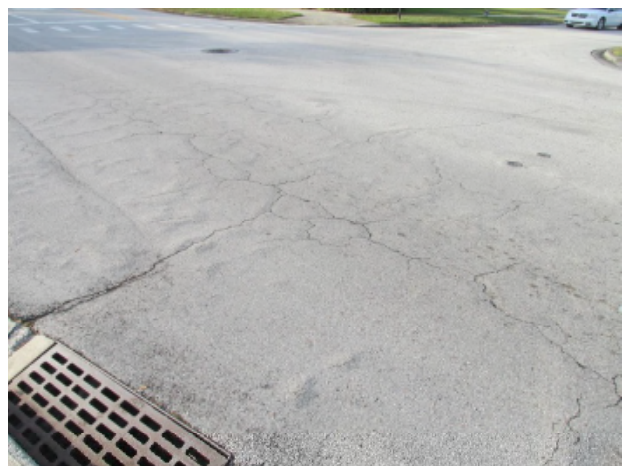
Asphalt pavement with alligator cracks and shoving
