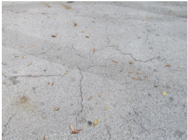
Asphalt pavement with alligator cracks
