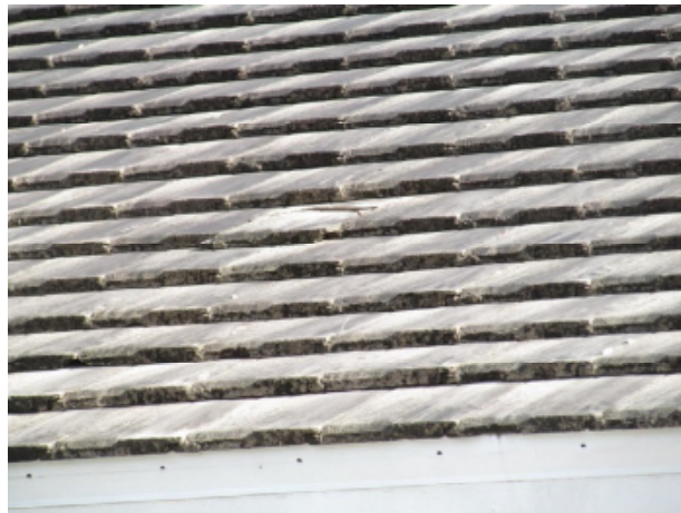
Concrete tile roof with broken tile
