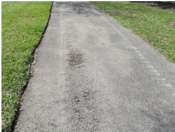
Asphalt walking path with surface deterioration
