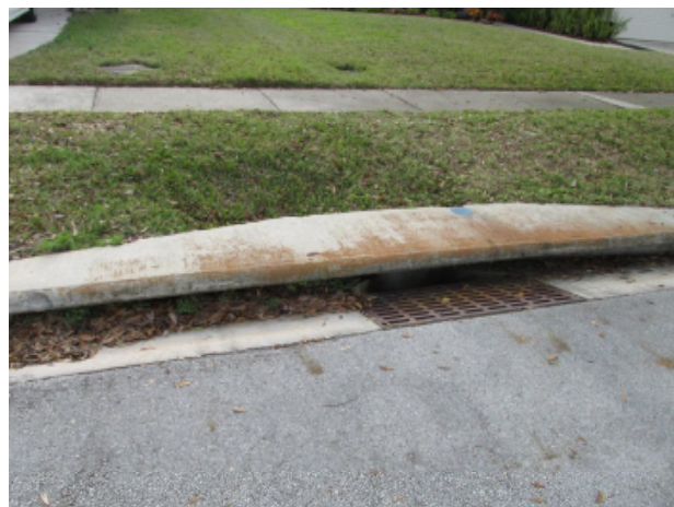
Severe settlement behind catch basin
