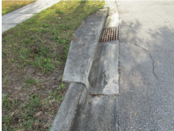
Severe settlement behind catch basin
