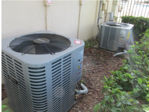
Condensing units for split systems
