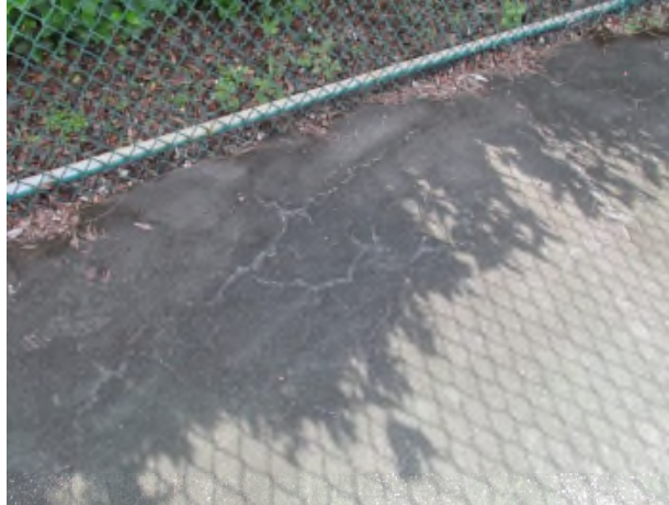
Hairline cracks evident
