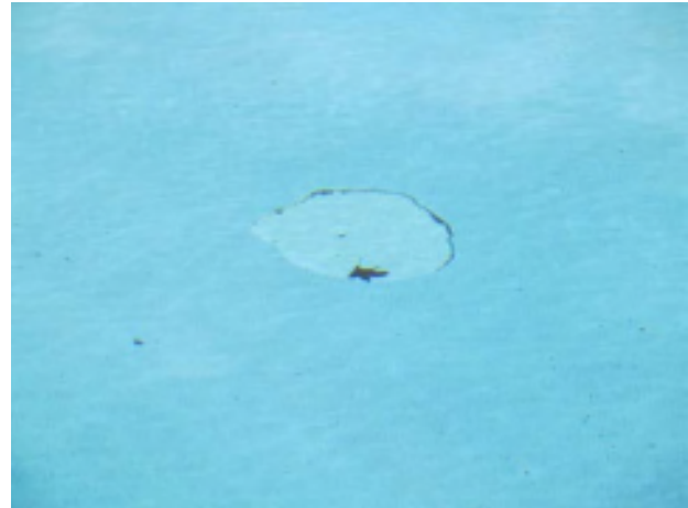
Missing plaster evident
