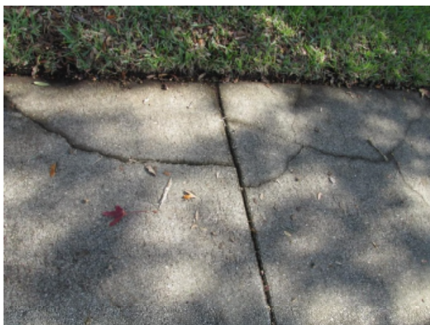
Concrete sidewalk with cracks
