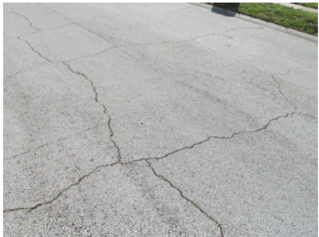
Asphalt pavement with block cracks
