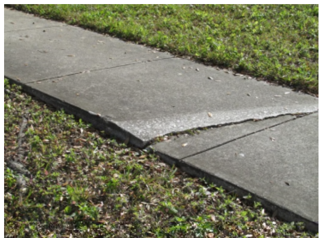
Concrete sidewalk with cracks and trip hazard
