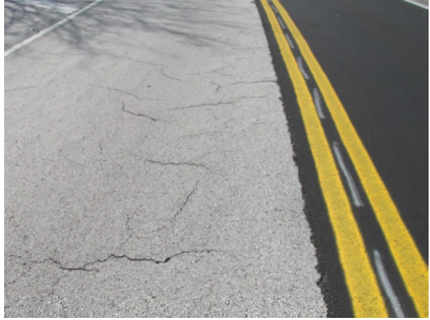
Asphalt pavement with slippage cracks
