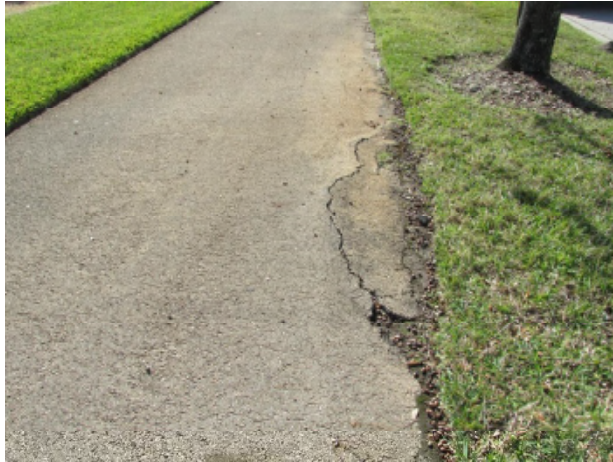
Asphalt pavement walkway with edge cracks
