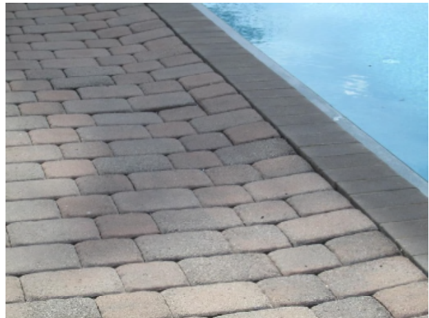
Deck pavers with isolated settlement evident
