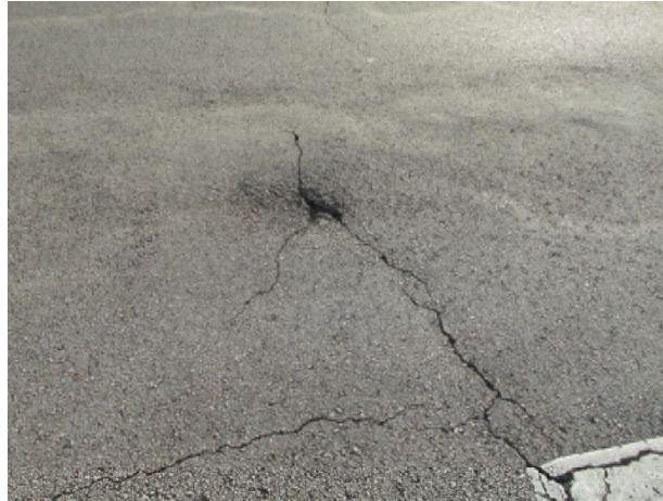
Asphalt pavement with pot hole
