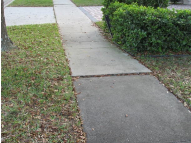
Concrete sidewalk with trip hazard
