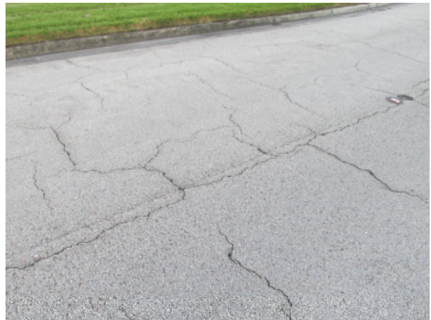
Asphalt pavement with severe block cracks
