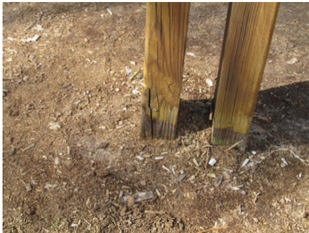
Playground equipment at clubhouse with isolated split wood evident
