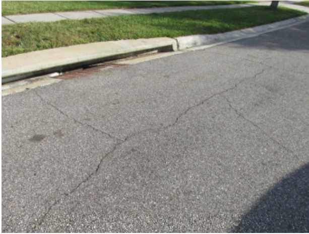
Asphalt pavement with block cracks
