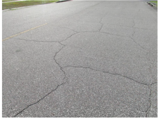
Asphalt pavement with block cracks
