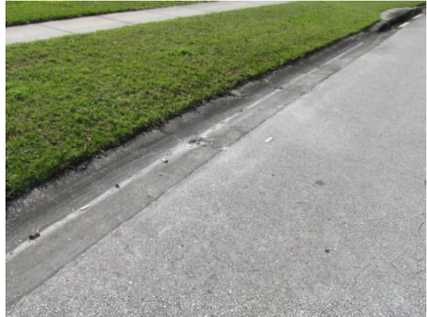
Concrete gutter with cracks
